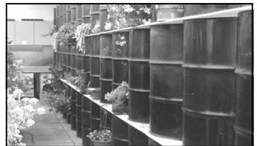
Barrels full of water that are one component of passive solar heating
